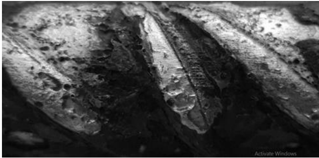
Fig.8. Cavities and deterioration on the ribs and deformations
