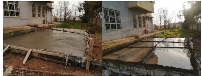
Figure (5) casting the concrete slab procedure
